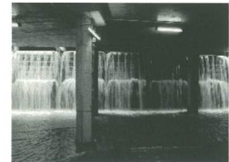
Figure 1: Happy Valley Underground Stormwater Storage Scheme: movable weirs
